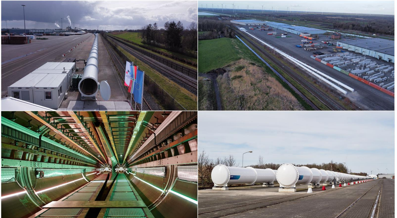
Figure 17: Test track at European Hyperloop Center
